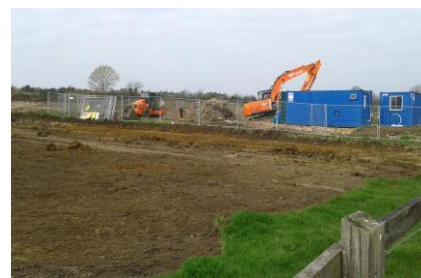
Groundworks for new housing to south of Grange Road, March 2019
